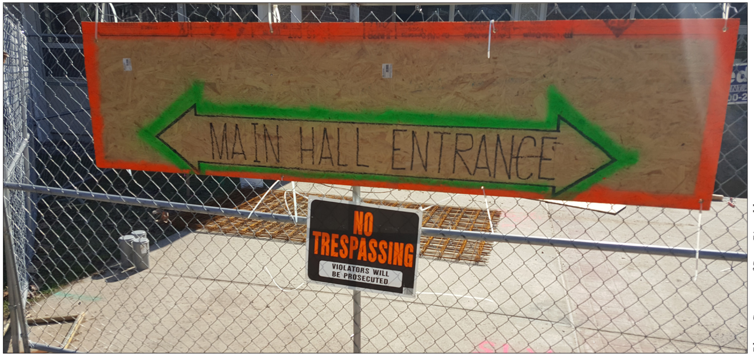
Main Hall, one of the busiest areas on campus, is having repairs.
